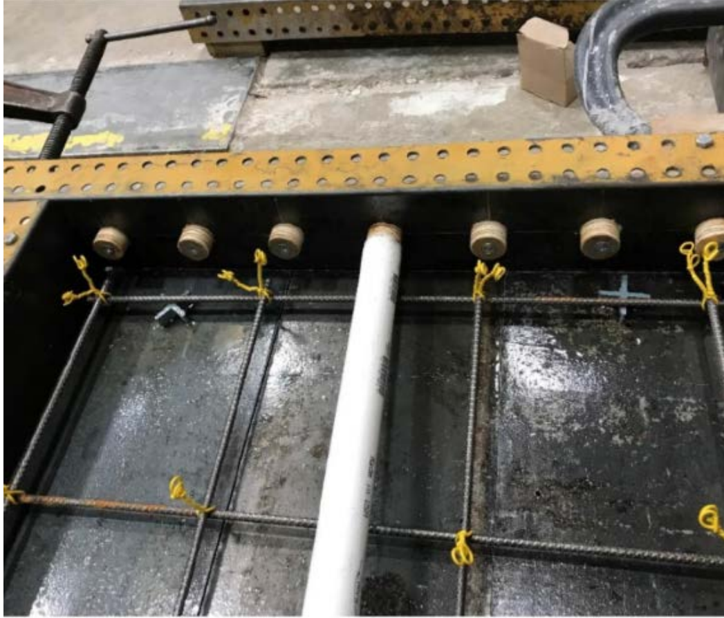
Figure 3-4. Construction of wall with embedded PVC tubes.
