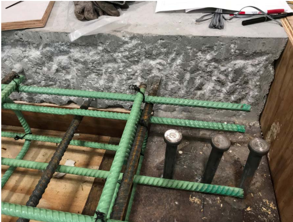
Figure 2-13. Construction joint at interface of existing bridge deck and concrete diaphragm sections.
