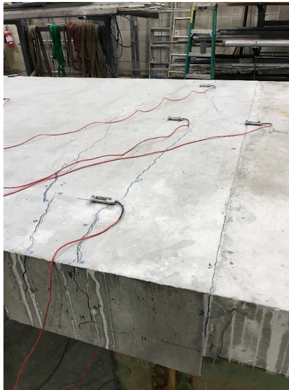
Figure 2-20. Crack at construction joint.
